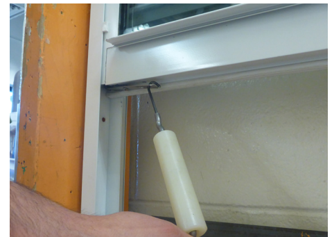
6. Using a hook, grab the bracket from the empty screw hole.
