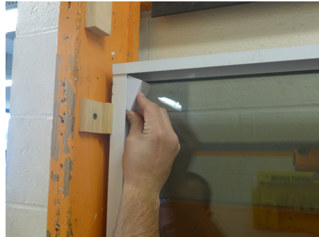
20. Replace top stops. Raise and lower sash to ensure proper operation.
