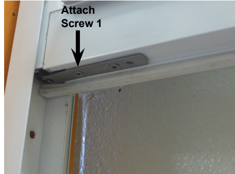
17. Insert screw 1 into the bracket.
