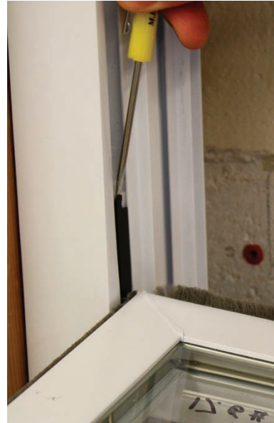
Step 6: Insert screw driver behind the top of the tamperlock
