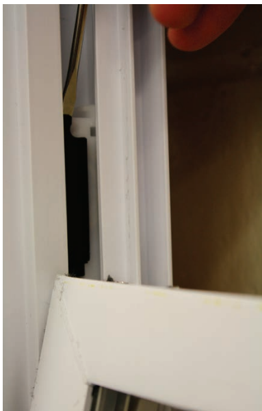
Step 16: Insert screw driver behind the top of the tamperlock. Pry top of tamperlock to disengage from opening.
