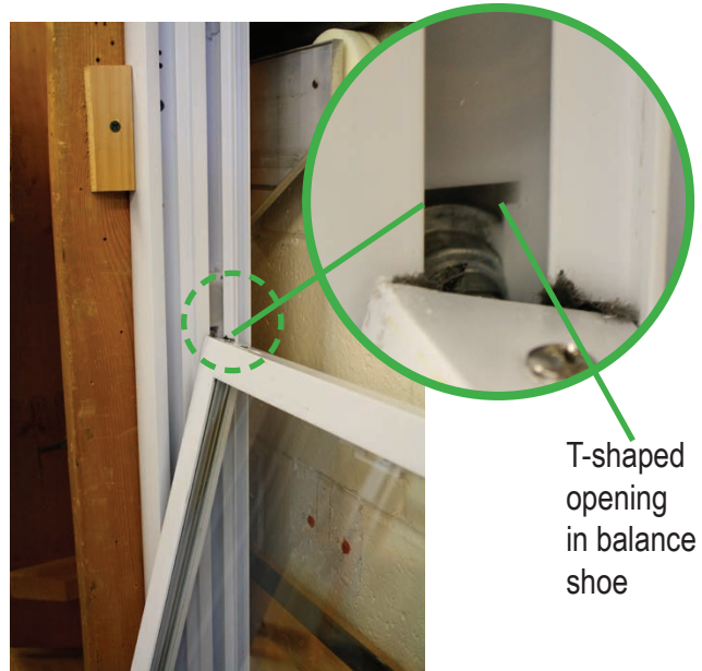
Step 24: Fully tilt sash down until T-shaped opening in balance shoe is completely visible.
