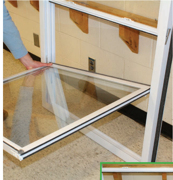
Step 10: Continue to push lower sash down until tamperlock is completely visible on the opposite side.
