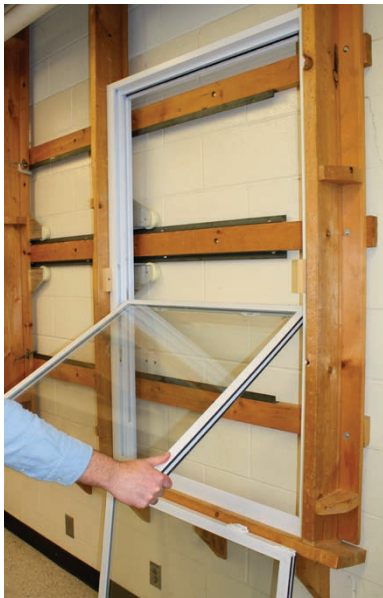
Step 14: Tilt upper sash down.
