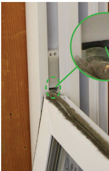
Step 34: Fully tilt sash down until T-shaped opening in balance shoe is completely visible.
