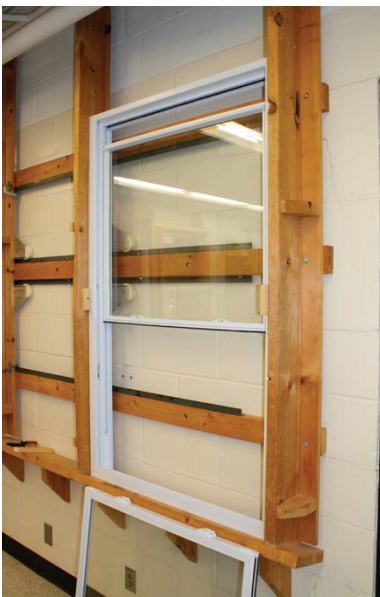
Step 12: Open the upper sash approx 1 inch.
