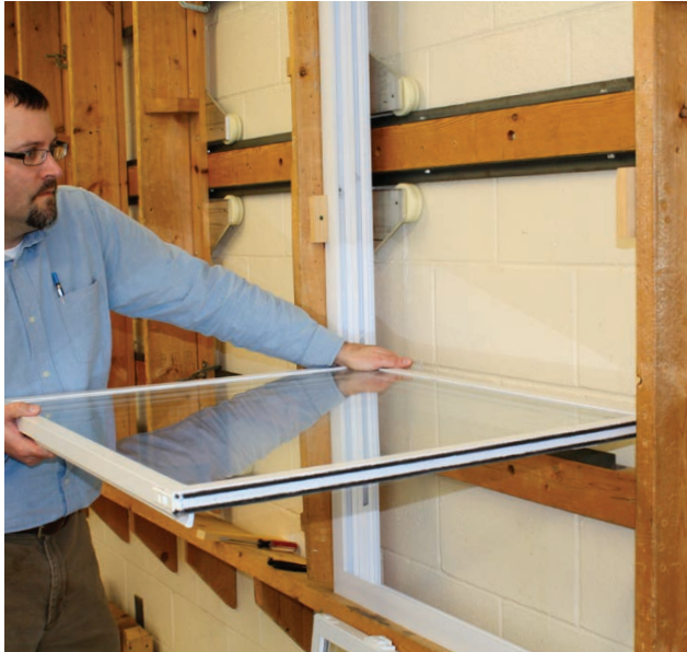
Step 23: Level sash by pushing down on highest sash corner near frame.
