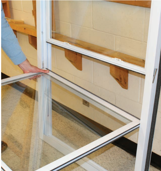
Step 9: Push down on lower sash near the window frame on the side that the tamperlock was removed.
