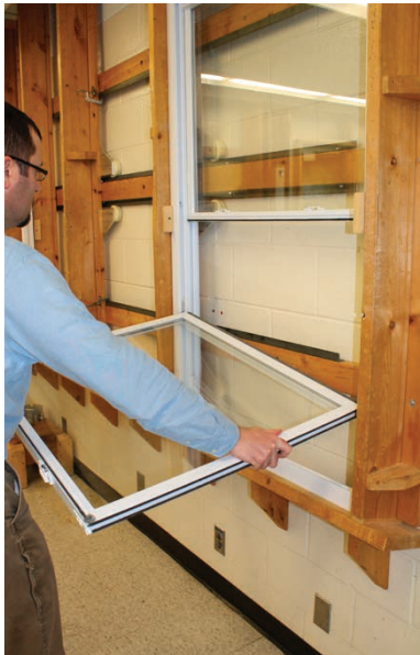
Step 32: Engage the sash pivot pin into balance shoes (See Steps 21 & 22)
