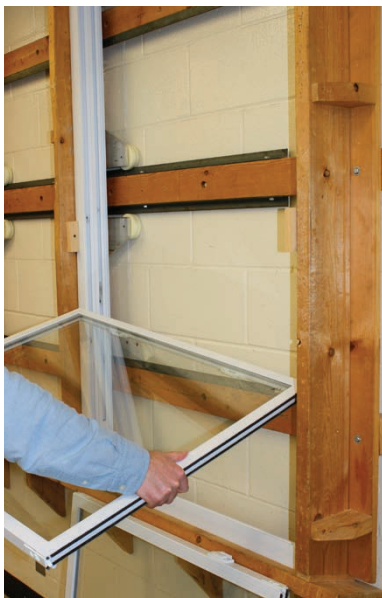
Step 21: Insert the upper sash. Engage first pivot pin into balance shoe.
