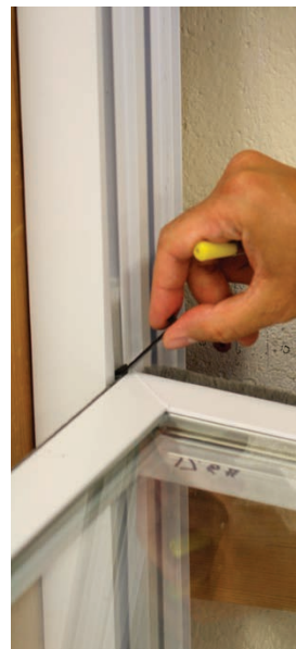
Step 8: Remove tamperlock from balance shoe by tilting towards the center of the window opening.
