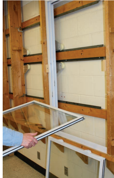
Step 20: Remove upper sash.
