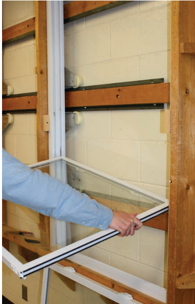
Step 19: Push down on the right or left side of the sash near the window frame until sash pivot pin on opposite side may be removed from balance shoe.
