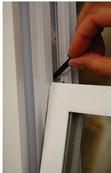
Step 26: Insert the tamperlock at an angle into the T-shaped opening indicated in Step 24.
