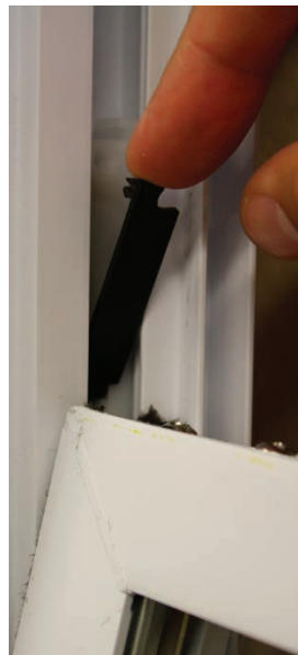
Step 17: Remove tamperlock from balance by tilting towards the center of the window opening.
