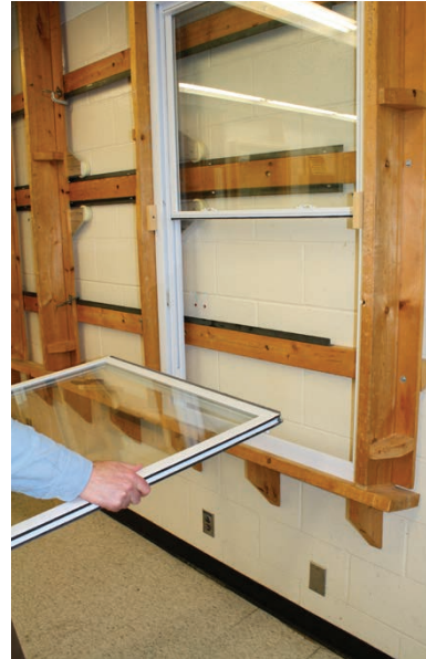
Step 11: Remove lower sash.
