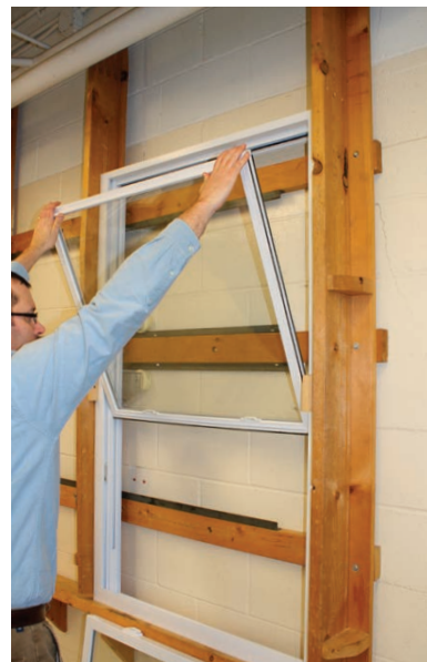
Step 13: Disengage tilt latches to tilt upper sash.
