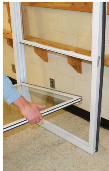
Step 12: Remove lower sash.
