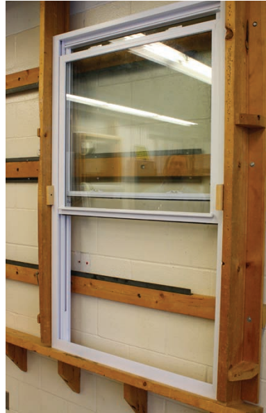
Step 2: Fully raise lower sash.
