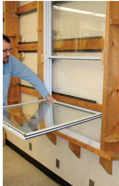
Step 33: Level sash by pushing down on highest sash corner near frame.
