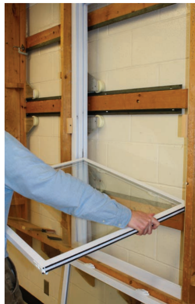
Step 22: Engage second sash pivot pin on opposite side into balance shoe.
