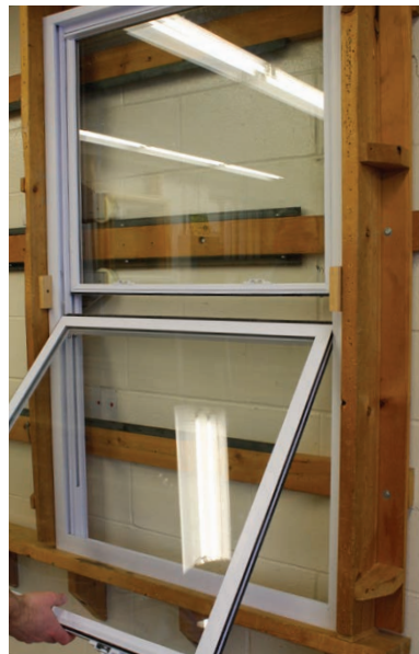
Step 4: Tilt lower sash down.
