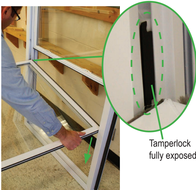
Step 5: Push down on the right or left side of lower sash near the window frame until tamperlock is completely visible on the opposite side.
