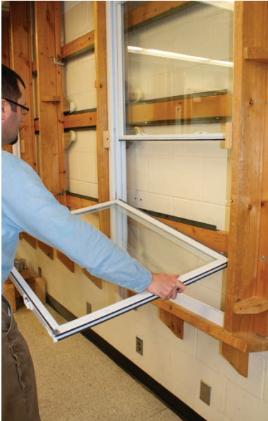
Step 10: Push down on the right or left side of the sash near the window frame until sash pivot pin on opposite side may be removed from balance shoe.
