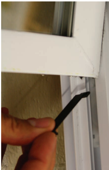
Step 25: Hold the tamperlock.
